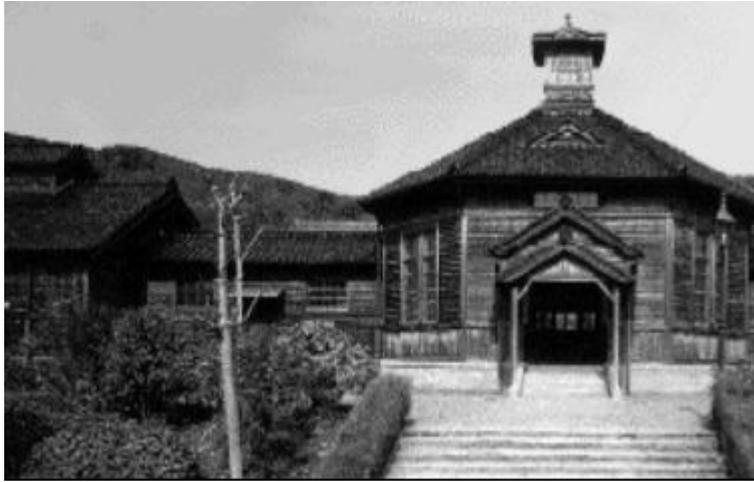
*Figure 3.5 Kanazawa Prison, constructed 1907, designed by Japanese architect, Yamashita Keijiro. Note the wooden construction, distinctive roof-style and octagonal central guard station from which five cell block radiate outward.<sup>65</sup>*
